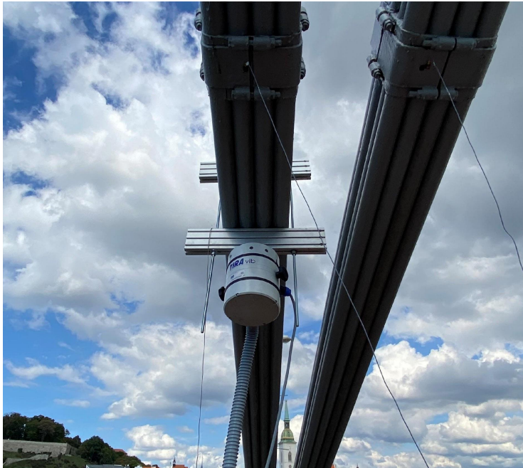
MODAL SHAKER on the CABLE 6
