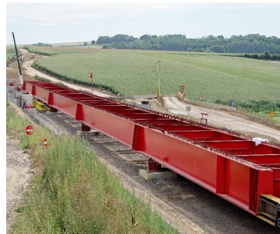
RAILVIADUC FOR HIGH SPEED TRAIN Rohrbach (France) – LGV Est
