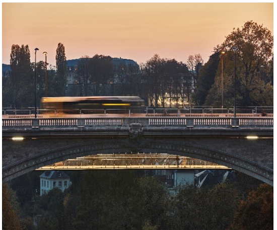
FOOTBRIDGE UNDER ADOLPHE'S BRIDGE Luxembourg-Centre
