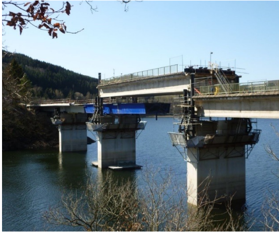
REPLACING ROAD DECK OA498 & OA499 Insenborn - Lultzhausen
